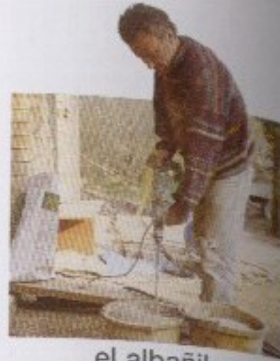
el albañil construction worker
