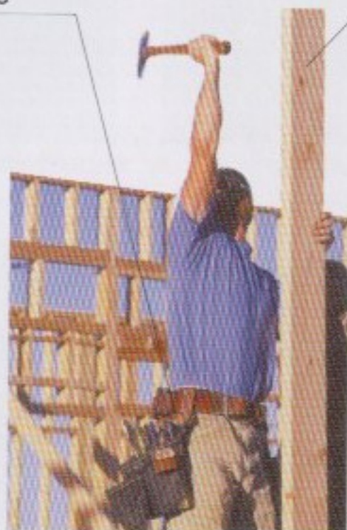
el albañil construction worker
